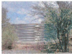
Open water reservoir (Source: Justin Johnson)
