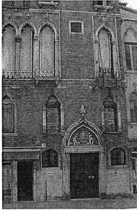
Figure 4: Example of a Lunetta on the Side of a Building in Castello
