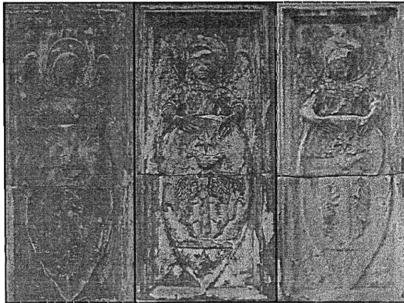
Figure 8: Example of Deterioration
