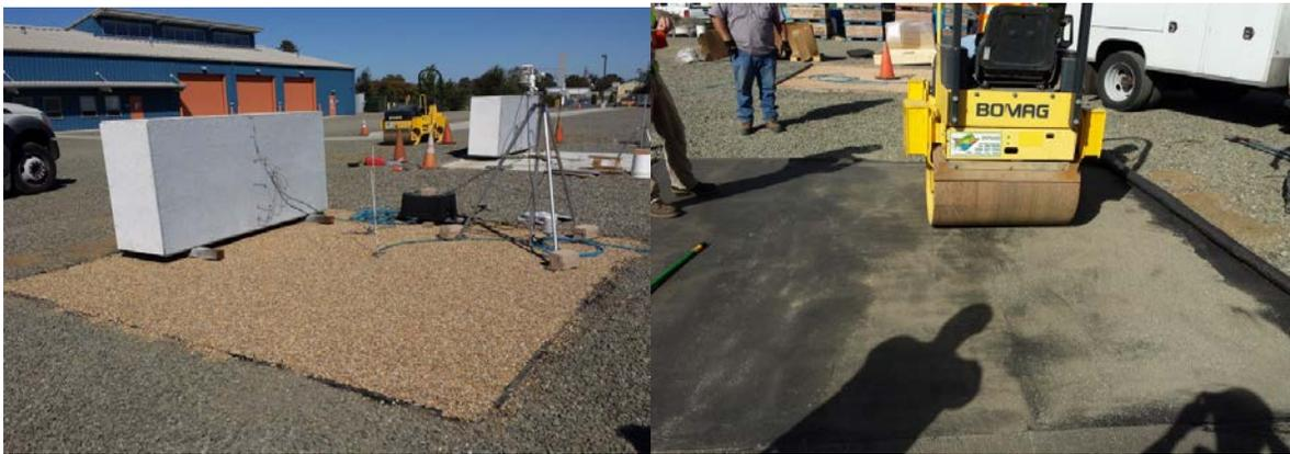
**Figure 7: GRCS at UC Davis Pavement Research Facility (completed left, rolling geosynthetic right)**
