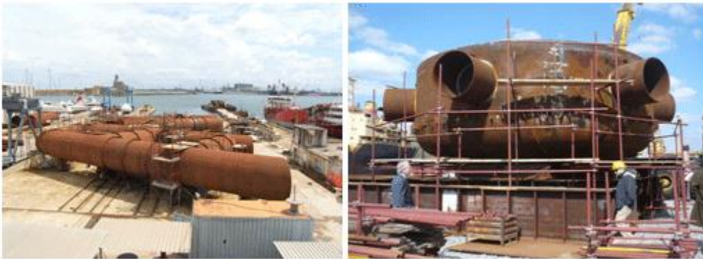
Figure 13 - Blue H TLP proof-of-concept currently under construction 24
