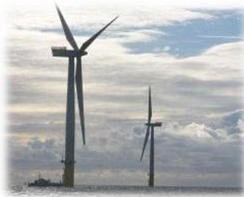
Figure 10 - The Walney wind farm uses Siemens SWT 3.6 wind turbines with a 107m rotor diameter 21
