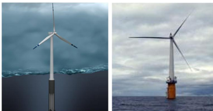
Figure 11 - Statoil hywind - computer model and full scale. The model shows the depth of the platform below the sea surface 22
