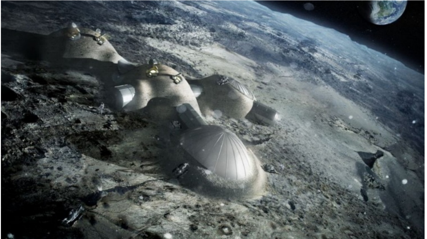
Figure 10: The top image showcases a render of a 3D printing robot placing layers of hardened lunar regolith on top of the inflatable dome shell. The bottom image displays a render of the completed lunar base design 81 .
