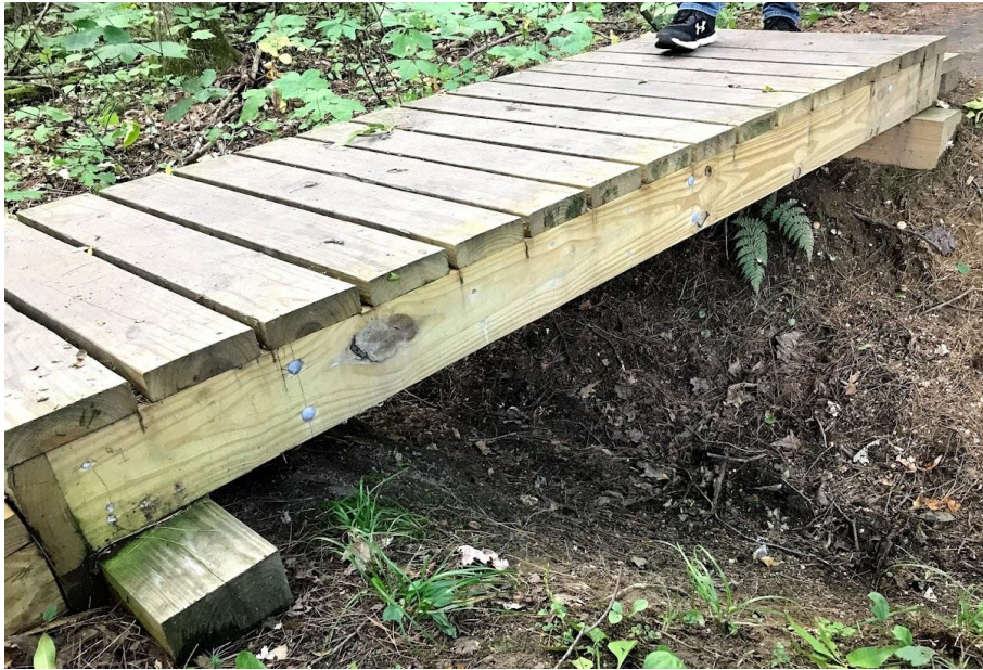
Bridge at Niquette Bay State Park
