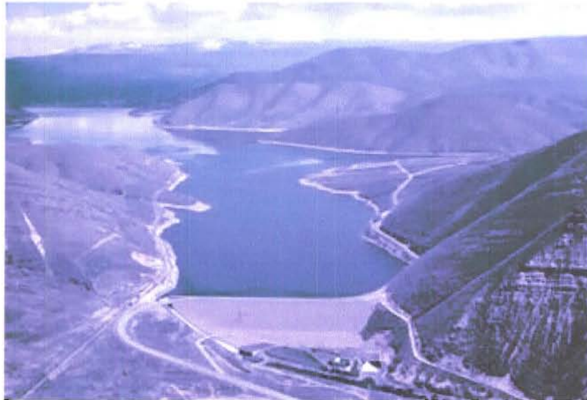
Figure 7: Deer Creek Dam and Reservoir ( http://www.usbr.gov/dataweb/assets/images/auto_generated_images/a_Deercrk.gif )
