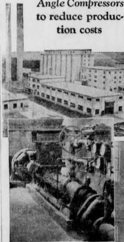
Two 1872-cu. ft. Balanced Angle Compound Compressors, direct connected to synchronous motors, in the plant of the Lawrence Portland Cement Company, Thomaston, Maine. They supply air for transporting cement, agitating clay and quarry drilling. View of the plant showing the 150,000-barrel silos; and the Fuller-Kinyon pumps.
