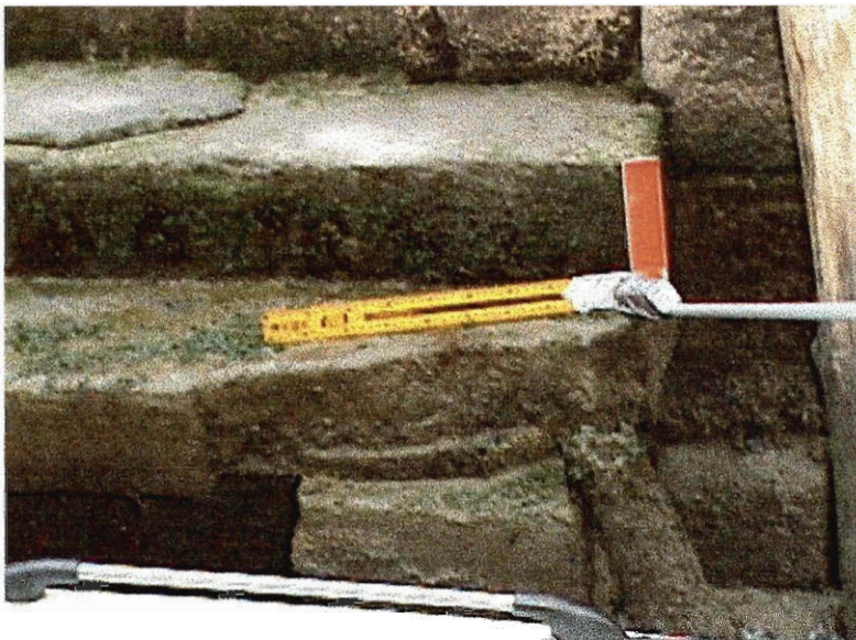
Figure 5-1 Image showing damage to istrian stone which is structural in origin and ruler used for reference
