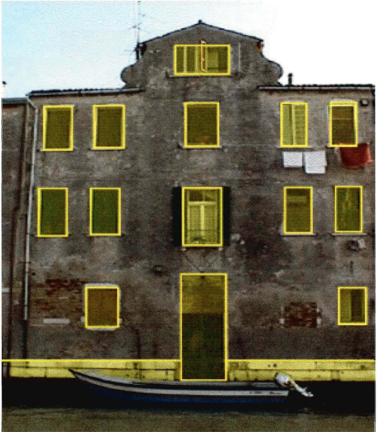
Figure 5-2 Diagram showing parameters for calculating quantity of plaster and estimated rate of deterioration
