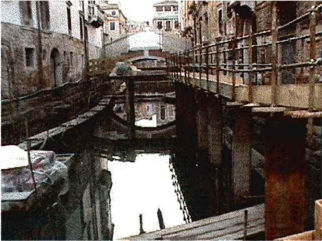
Figure 5-1 Image showing canal dredging in progress
