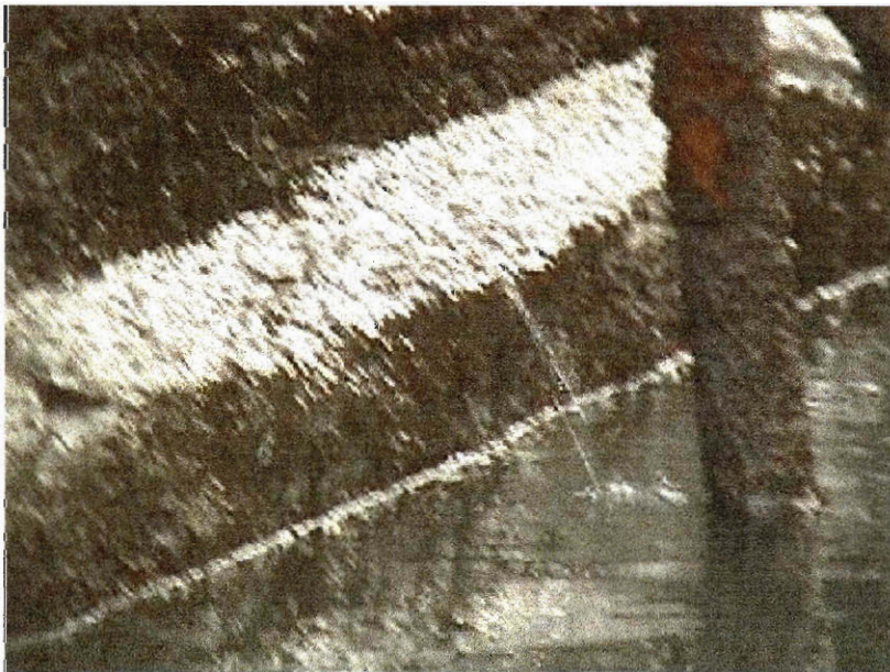
Figure 7-1 Image showing wastewater flowing from a crack in the canal wall which will cause further deterioration if not repaired
