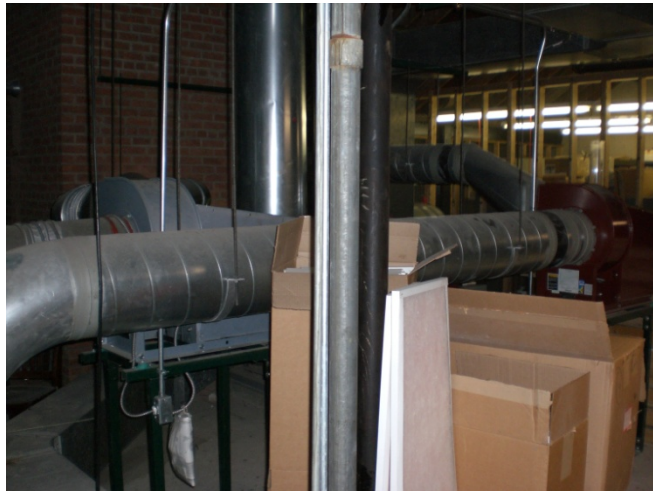
Figure 2.7 Primary Ventilation System
