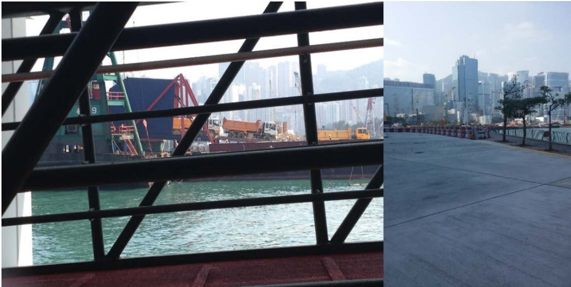
Figure H-47: Area in Wan Chai is under land reclamation
