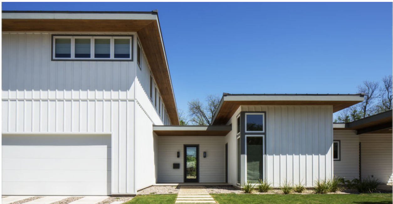
Figure 15 - James Hardie Panel Vertical Siding real world application
