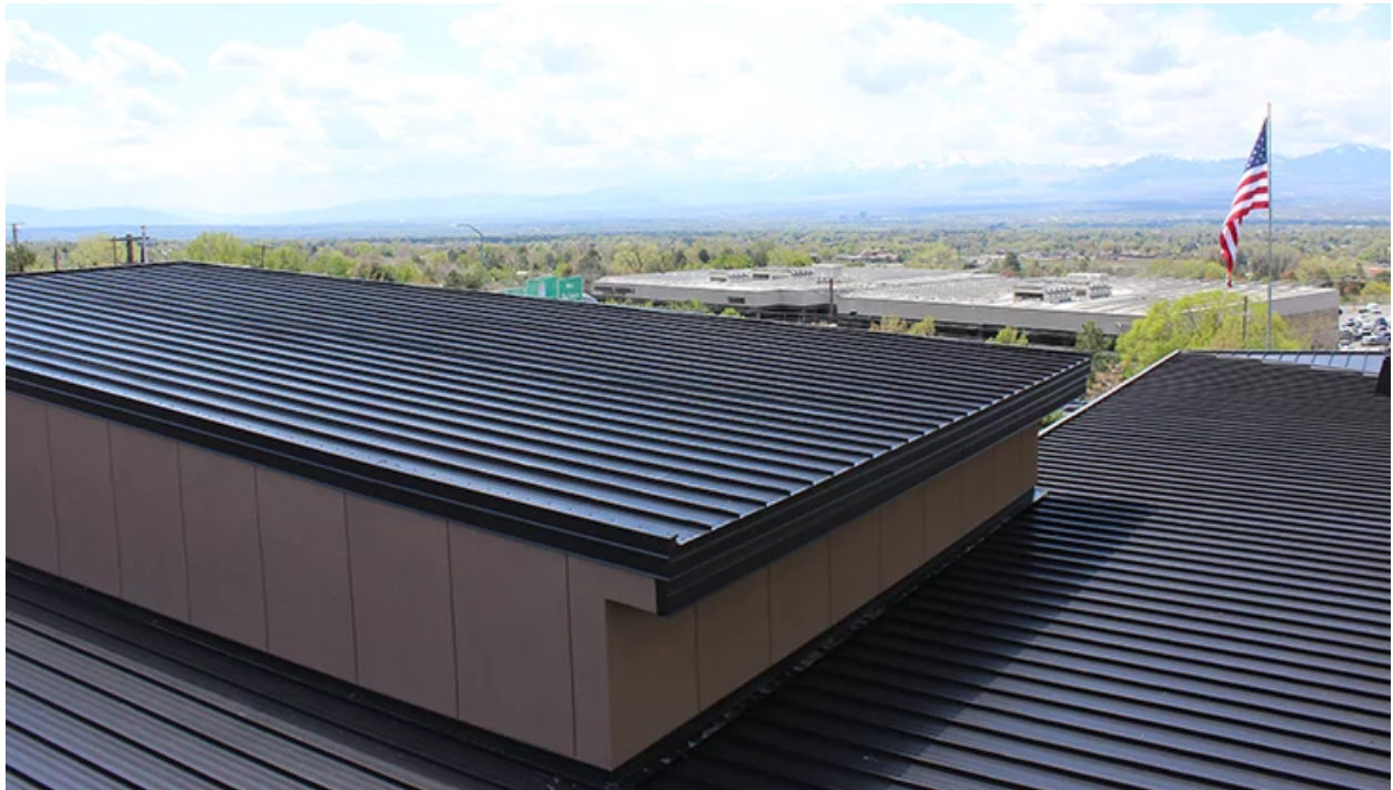
Figure 16 - MBCI Superlok® utilized on an assisted living building.
