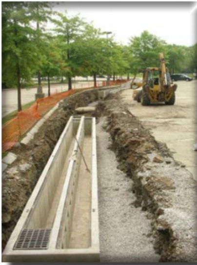
Figure 8: Sand & Organic Filter (Commonwealth of Massachusetts, 2018)
