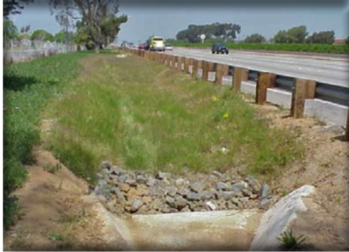
Figure 11: Grassed Channel (Commonwealth of Massachusetts, 2018)
