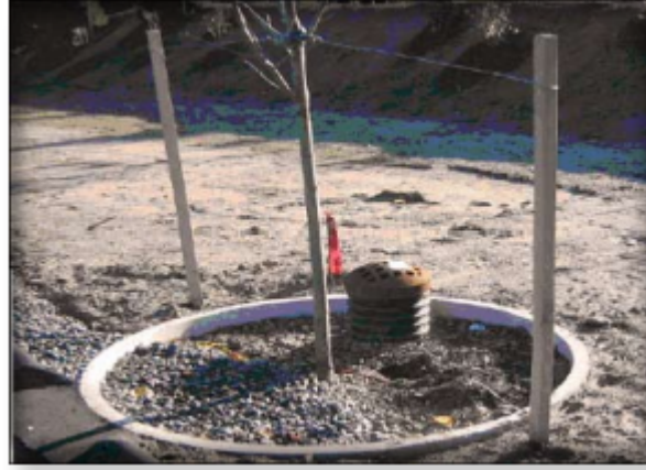
Figure 9: Treebox Filter (Commonwealth of Massachusetts, 2018)
