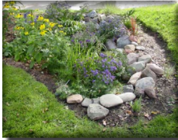
Figure 5: Bioretention Area/ Rain Garden (Commonwealth of Massachusetts, 2018)
