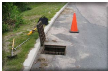
Figure 4: Leaching Catch Basin (Commonwealth of Massachusetts, 2018)
