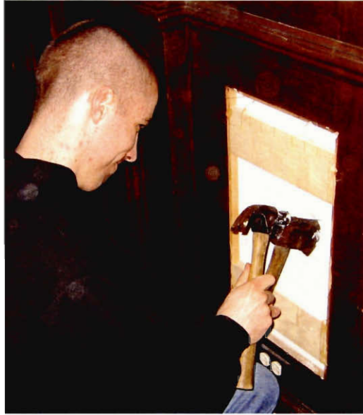
Fig. 3-35 Cutting Through the Wall in Spaulding
