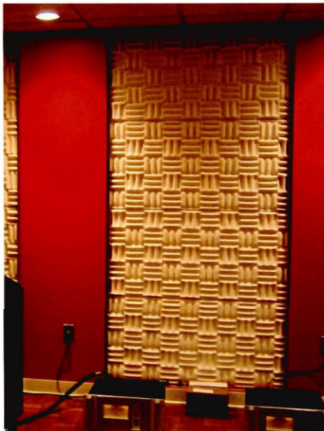
Fig. 2-7 Thick Absorptive Foam on the Wall
