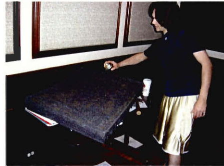
Fig. 3-25 Applying Foamtak to Foam Panel
