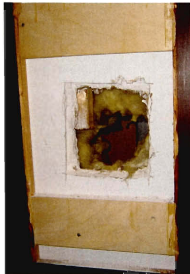
Fig. 3-36 Hole Before Insulation Removal
