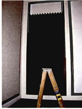
Fig. 3-24 Partially Completed Treatment
