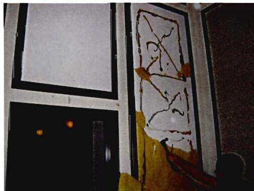
Fig. 3-21 Glued Panel Removal
