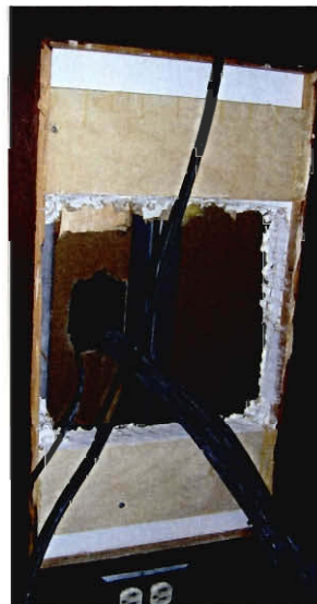
Fig. 3-37 Hole After Insulation Removal
