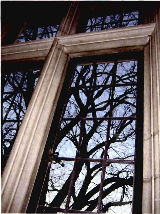
Fig. 3-4 Windows Facing West Street
