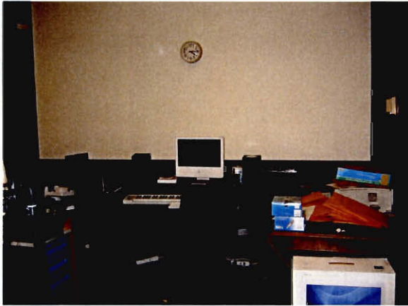
Fig. 3-19 North Wall of Control Room
