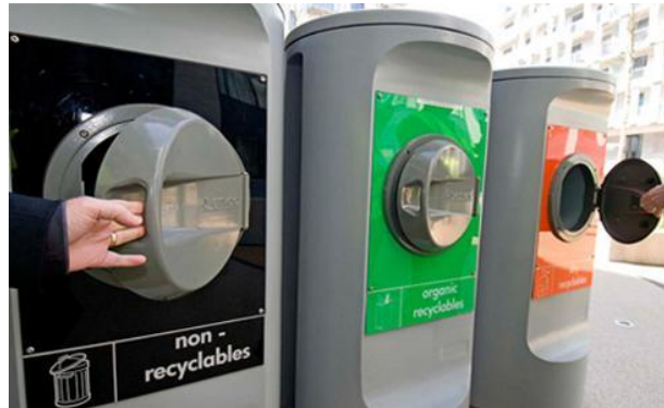
Figure 16: Envac Disposal System
