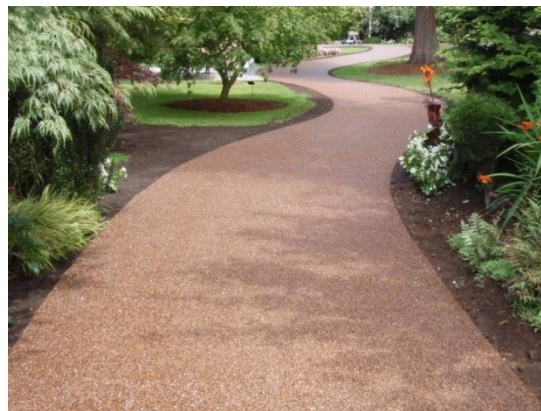
Figure 5. Filterpave for pedestrian walkway (Permeable Pavers, n.d.)
