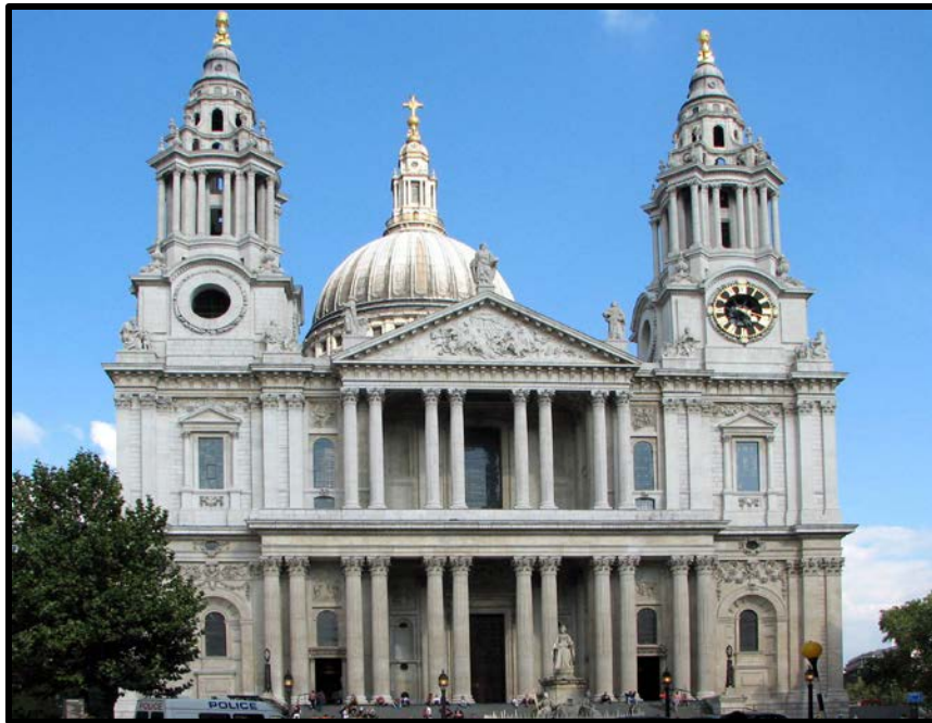
FIGURE 27: ST. PAUL'S CATHEDRAL ENTRANCE
