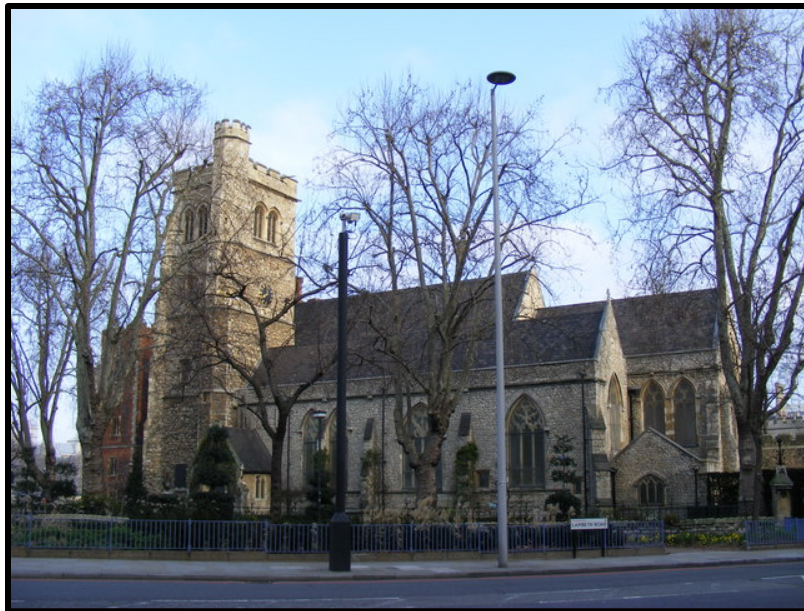
FIGURE 24: ST. MARY'S SIDE EXTERIOR
