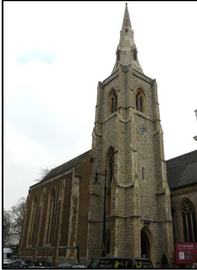
FIGURE 29: ST. MICHAEL, CHESTER SQUARE, EXTERIOR
