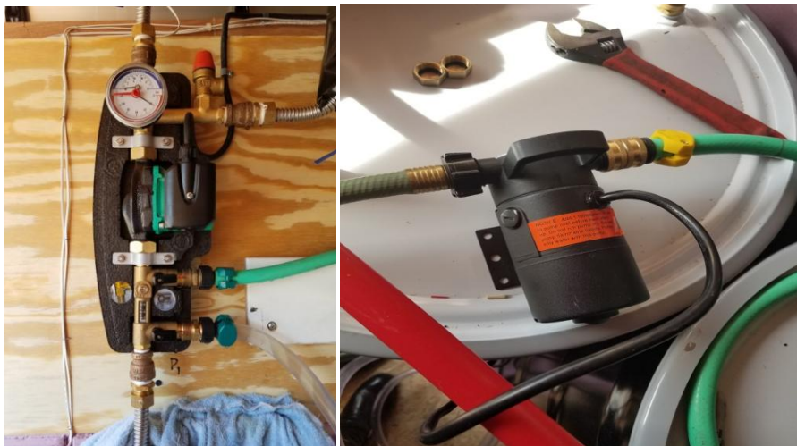
Figure 36: Attaching the Hose to the Wilo Star and Small Pumps
