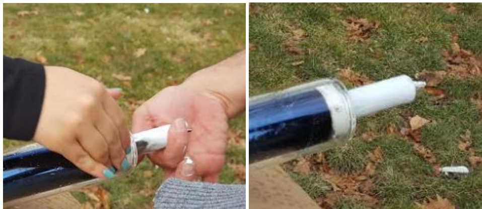
Figure 34: Applying Heat Transfer Paste and Soapy Water
