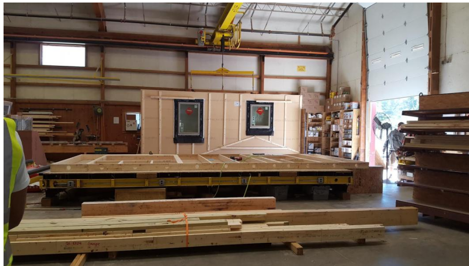
Figure 22: Wall Panels Being Assembled in Unity Homes' Factory
