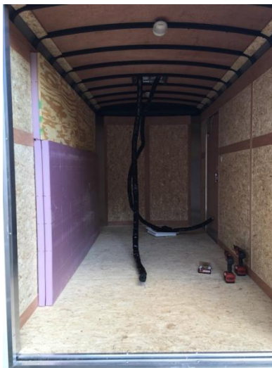
Figure 31: Insulating the Side of the Trailer
