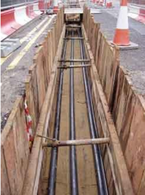
Figure 15: directly buried cable installation (EMFS, 2014)
