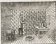
Registered Cellular Bins.
