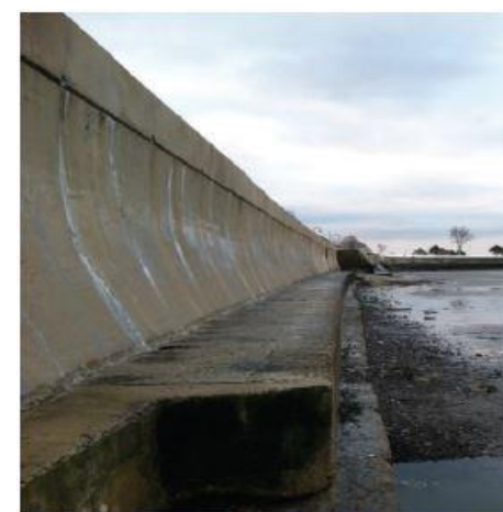
Figure 8: Implementation of a Seawall (Tinari, 2017)
