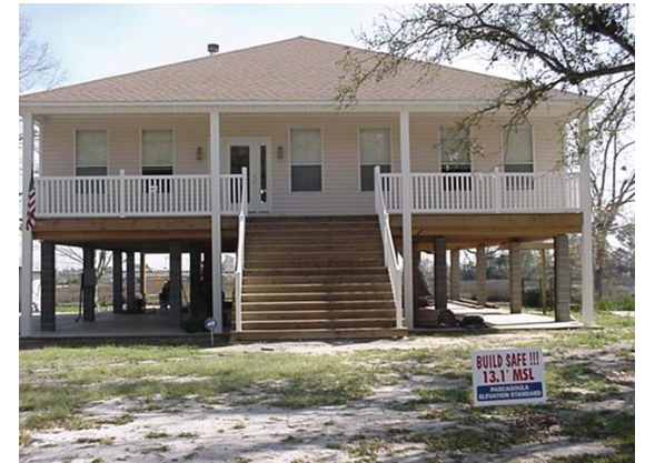
Figure 16: Raising Infrastructure (The U.S. National Archives, 2007)
