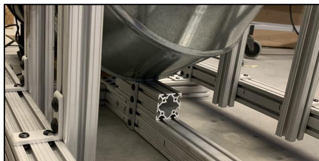
Figure 14: Bottom elbow duct support
