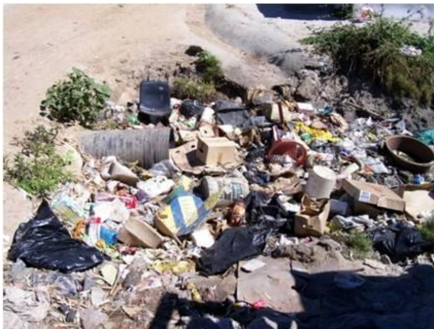
Figure 22: Blocked infrastructure in Phola Park Philippi
