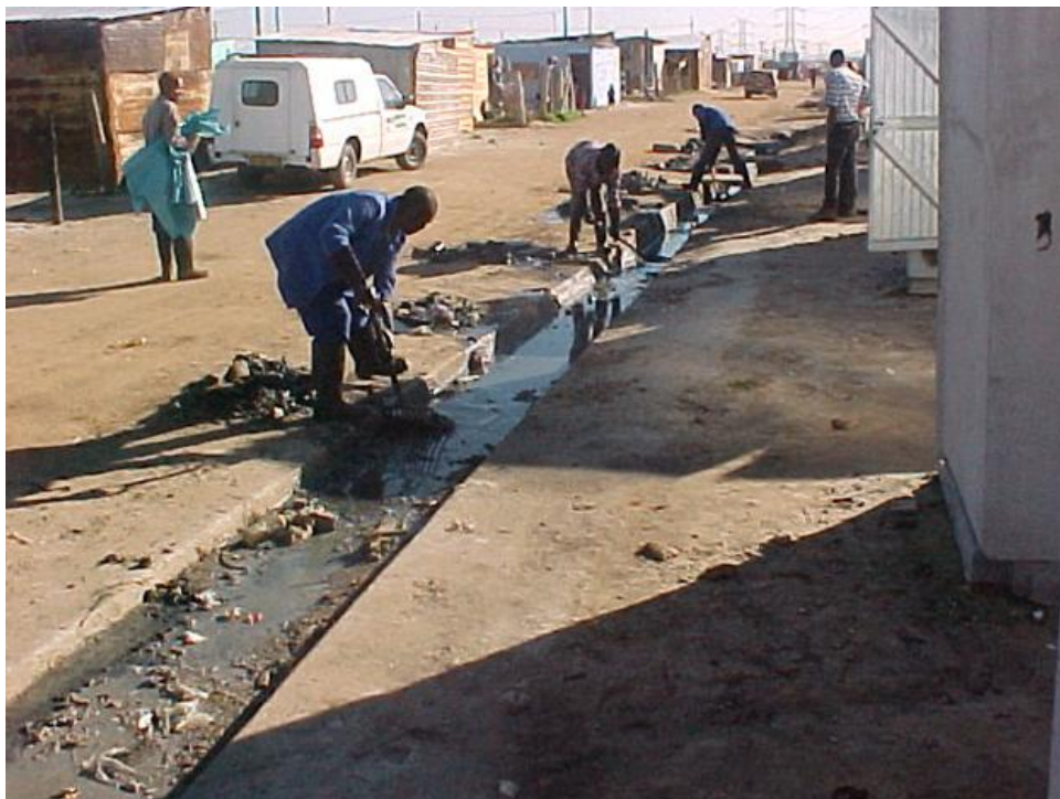
Figure 3: Stormwater infrastructure in the informal settlements
