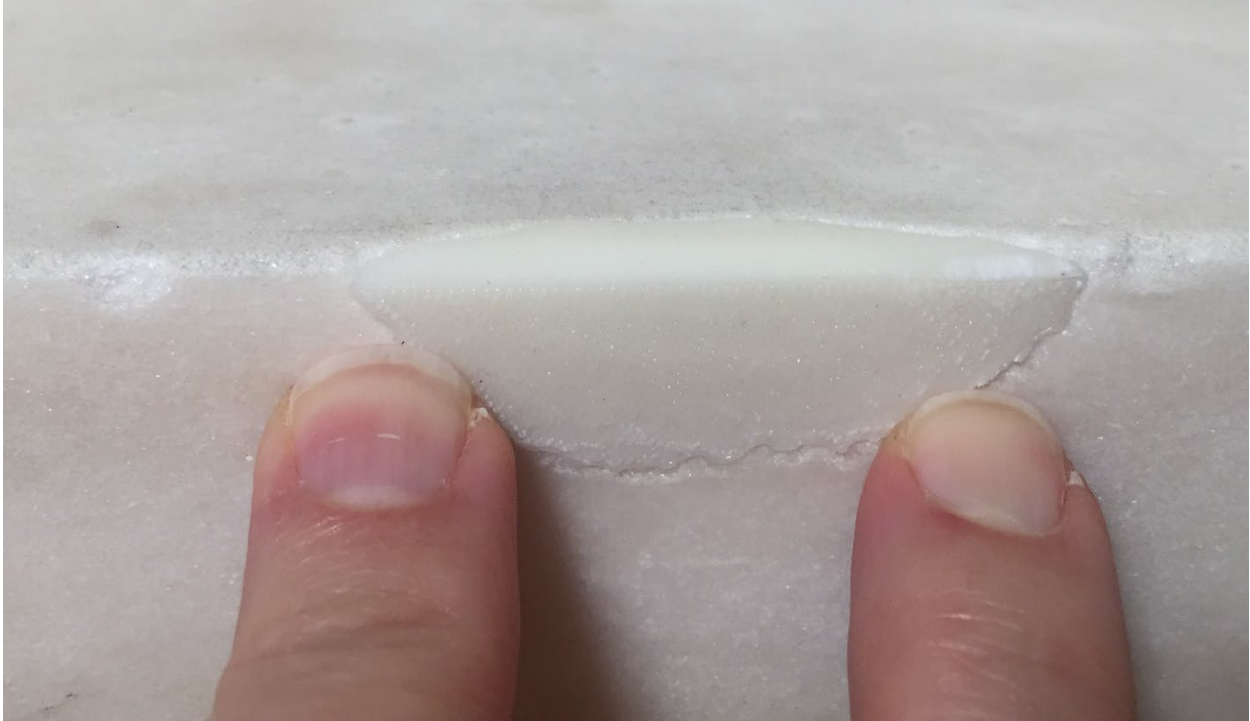
Figure 5.24: A printed piece cleanly filling in the missing portion of the pedestal
