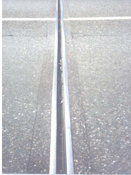
Figure 3: Strip Seal Joint ( Bridge Deck Joint Performance, 2003 )
