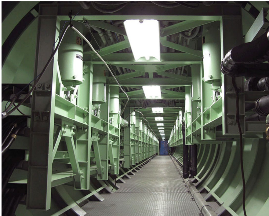
Titan II Missile Silo Hallway. Source: URL
