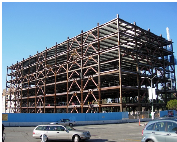
Figure 24: Example of a braced frame lateral system
