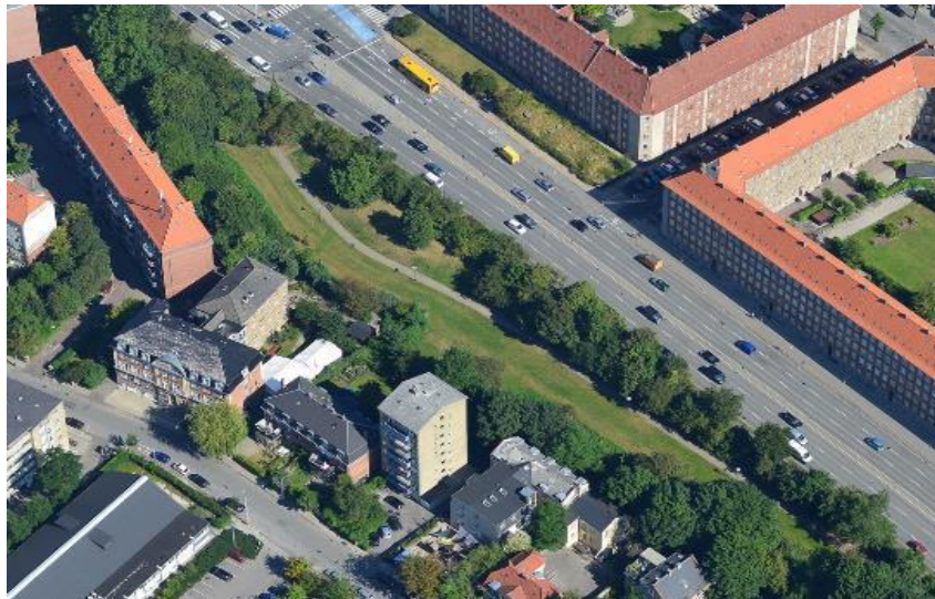
Figure 15: An aerial view of Ågadeparken (City of Copenhagen, 2015).
