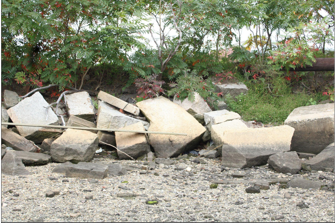
Figure 17: Bank that Separates the Shoreline Area from the Upland Area.
