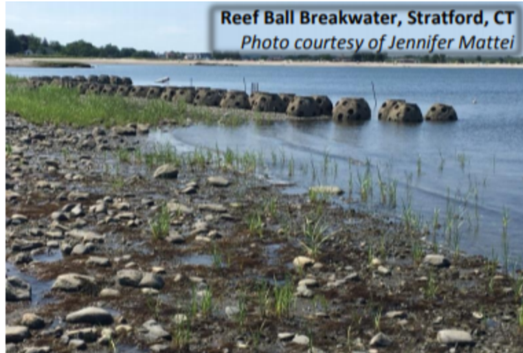
Figure 11: Reef Ball Breakwater in Stratford, Connecticut. ( Living Shorelines in New England , 2017)
