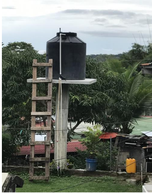
Figure 1: Water Tank in Burunga
