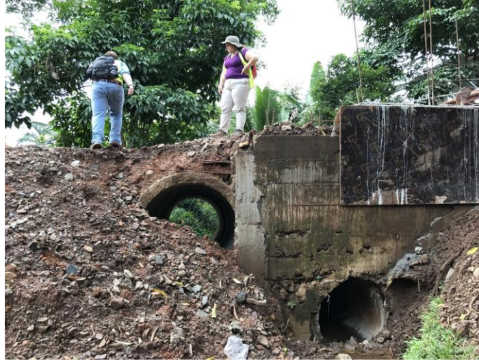
Figure 6: Measuring culverts in La Alameda
