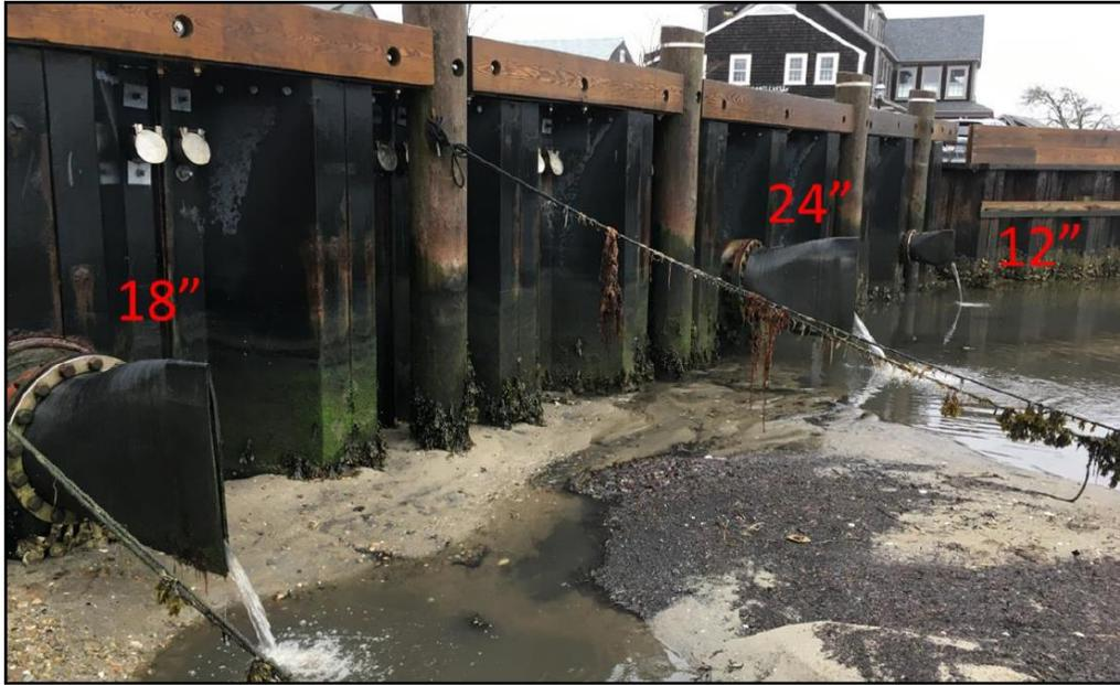
**Figure 9: Easy St. Bulkheads with sizes of the duckbills (Larson, *High-Tides and Flooding on Easy Street 2020*)**
