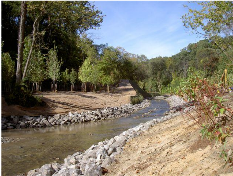
Figure 8 - Stream bank showing the use of riprap for erosion control (Michigan Department of Water Resources, 2011)
