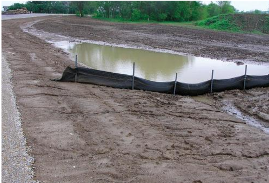
Figure 6 - A properly installed silt fence retaining run-off for sedimentation and filtration to occur (Carpenter, 2006)
