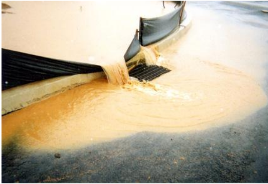
Figure 7 - Overlapping and collapse of a silt fence due to flooding when installed at a concentrated flow (Carpenter, 2006)
