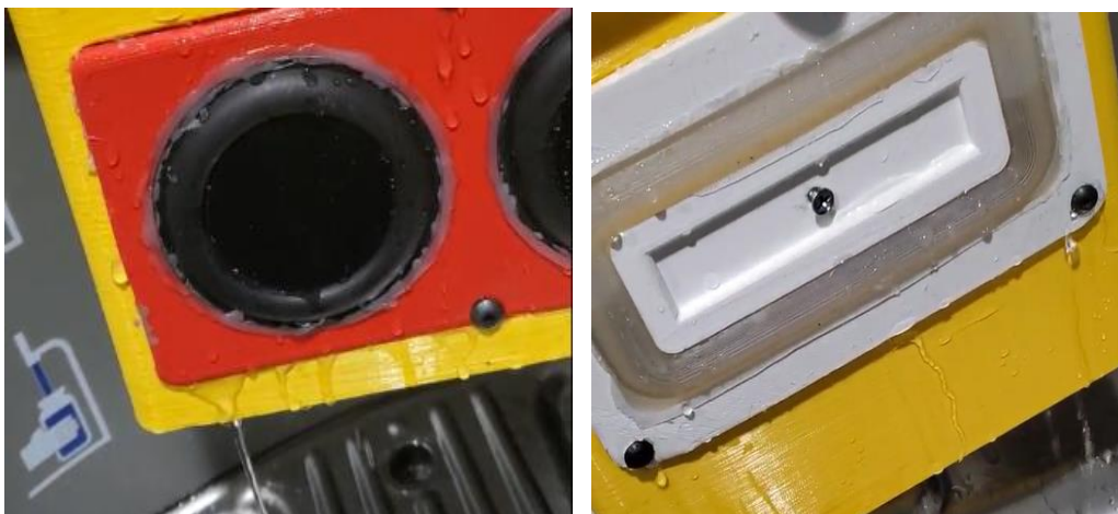
Figure 5: Water leaking from 2023 speaker from water test
