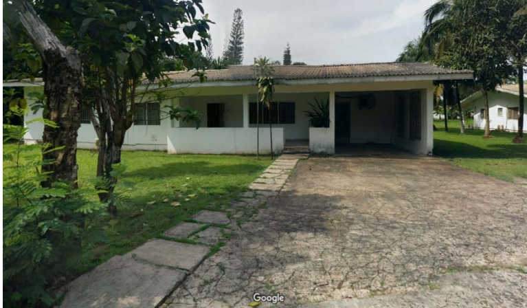
Figure 10: Home in Liberia with Corrugated Roof
