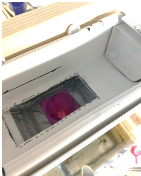
Figure 24: Funnels Placed on Top of Downspout
