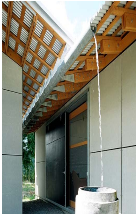
Figure 21: Open End Gutter
