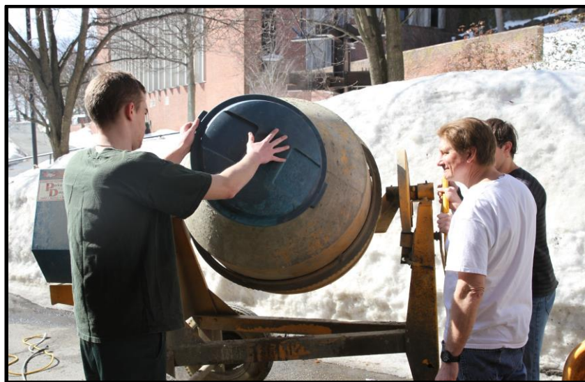
Figure 17: Concrete Mixing. From Kaven Hall, Worcester Polytechnic Institute (3/11/2015). Photo by Dan Sanderson.
