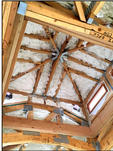
Figure 4.6 Blown-in foam insulation used in a cupola (Sanders, 2017)
