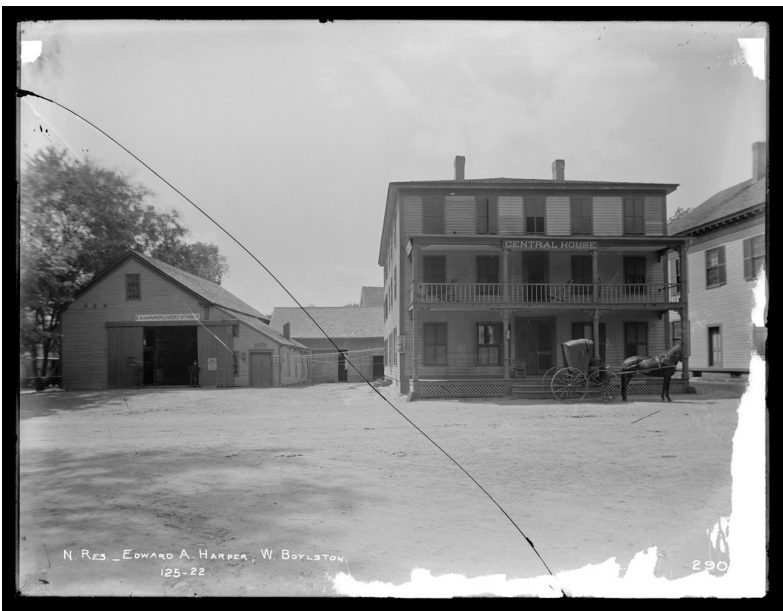
Figure 58: Edward Harper's Central House and Stable
