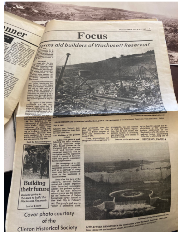
Figure 23: Article Detailing the Construction
