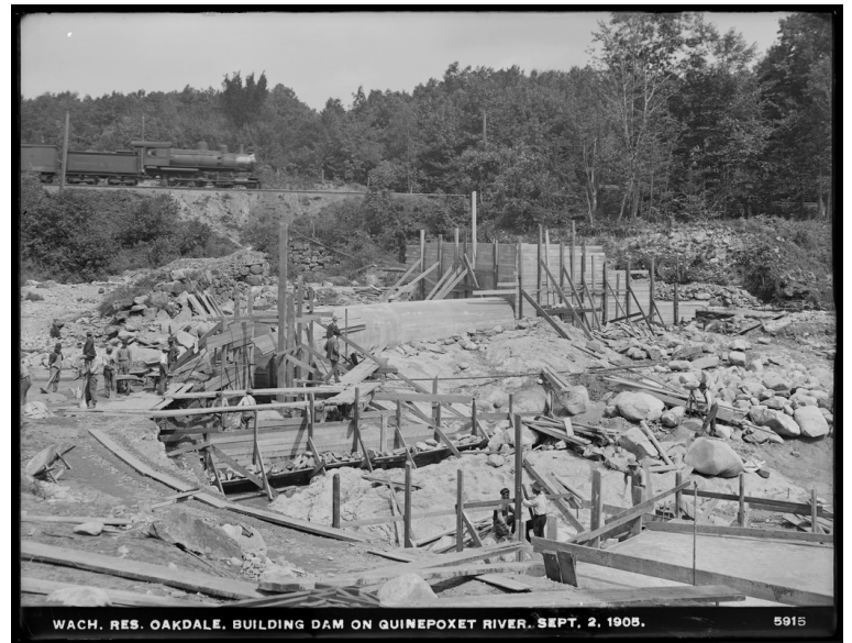
Figure 27: Construction of Wachusett Reservoir 14
