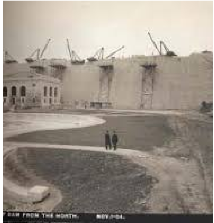
Figure 14: Wachusett Reservoir Construction 14
