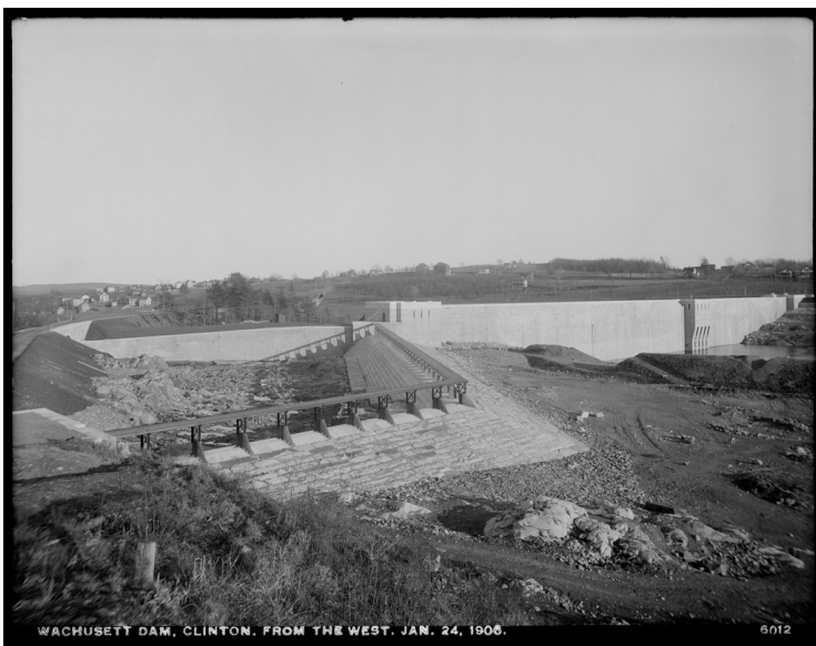
Figure 15: Wachusett Reservoir Construction 14
