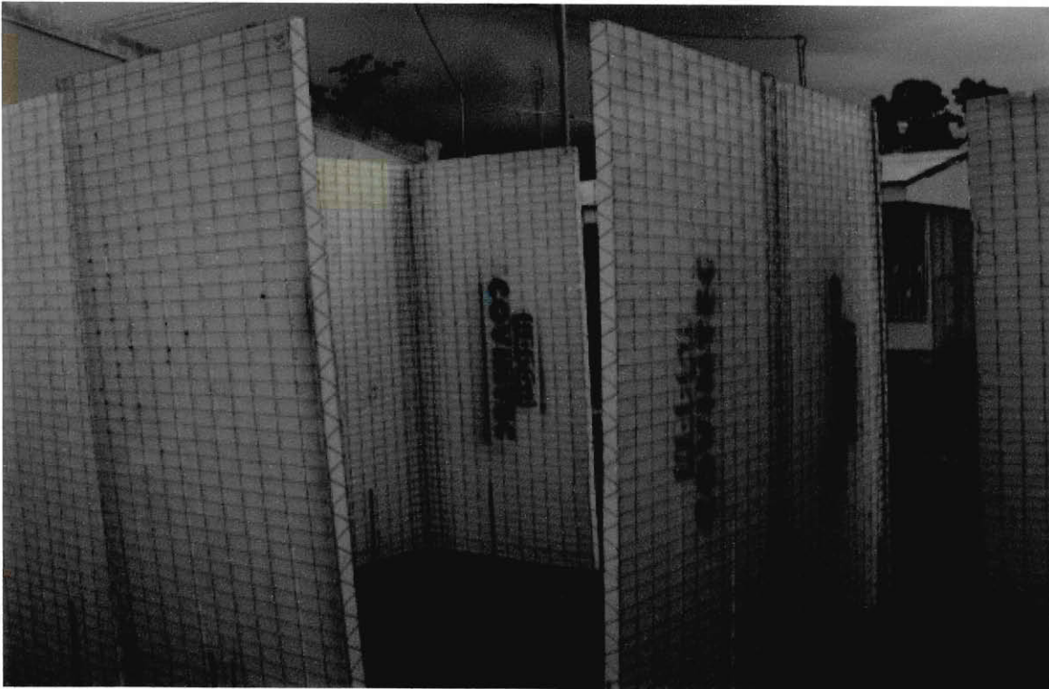
WALL BEING CONSTRUCTED WITH COVINTEC PANELS
