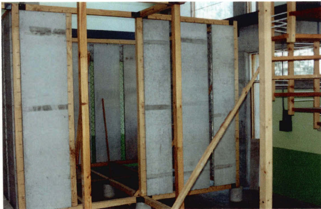
HABICON WALL PRIOR TO FINAL MORTAR
