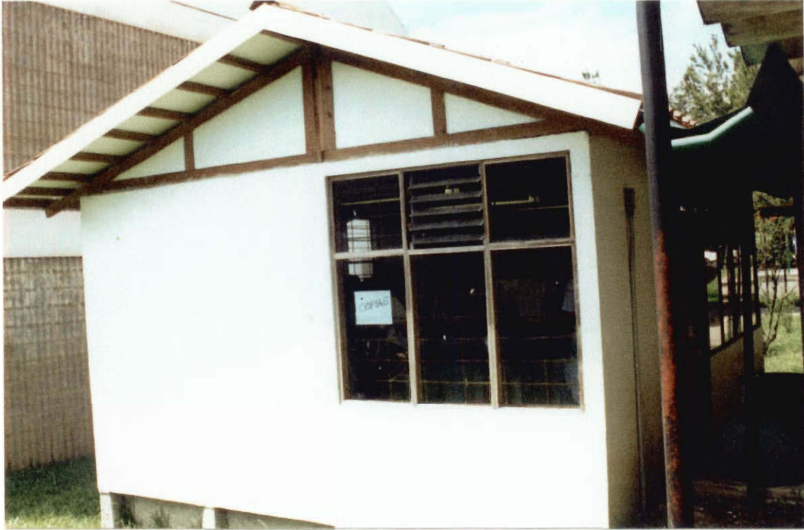
FINISHED HOUSE MADE ENTIRELY WITH THE HABICON SYSTEM
