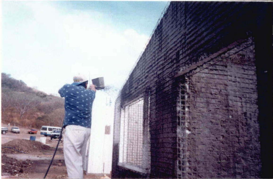
ROUGH MORTAR BEING APPLIED TO WALL USING MORTAR GUN
