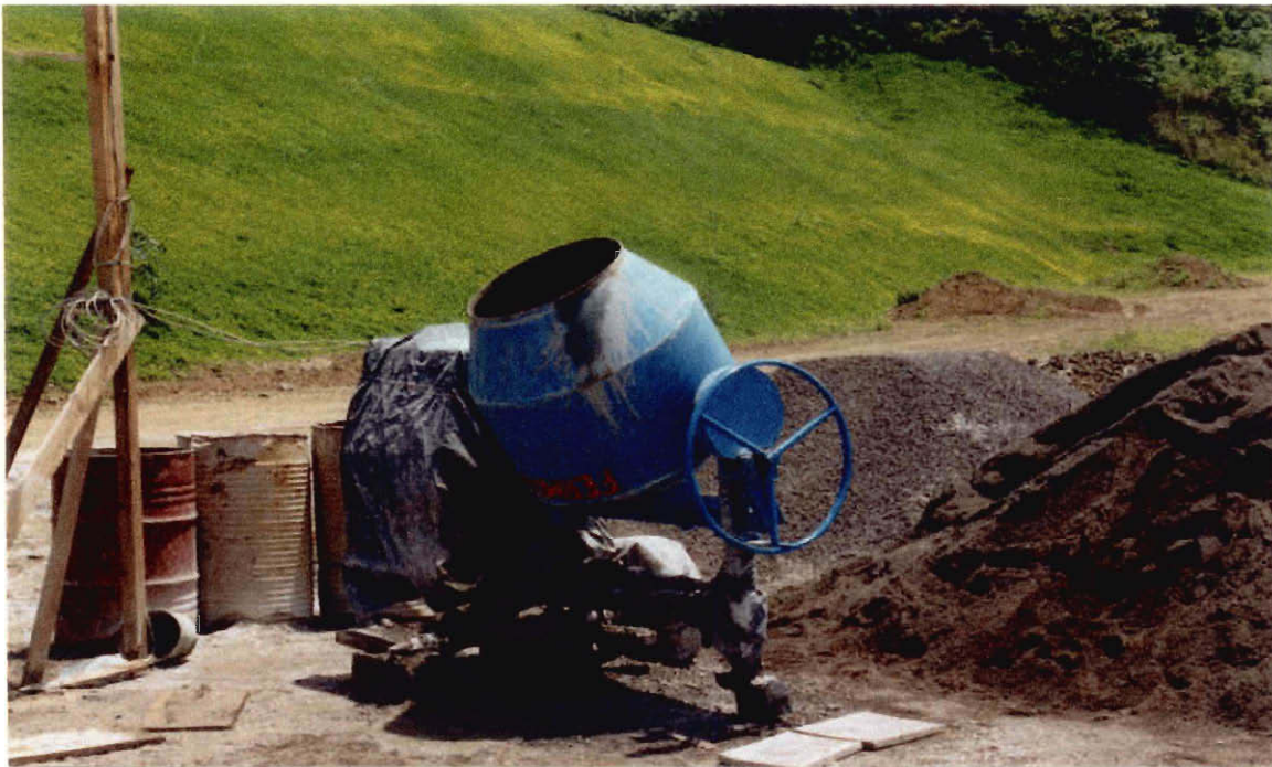
CEMENT MIXER USED FOR MIXING MORTAR
