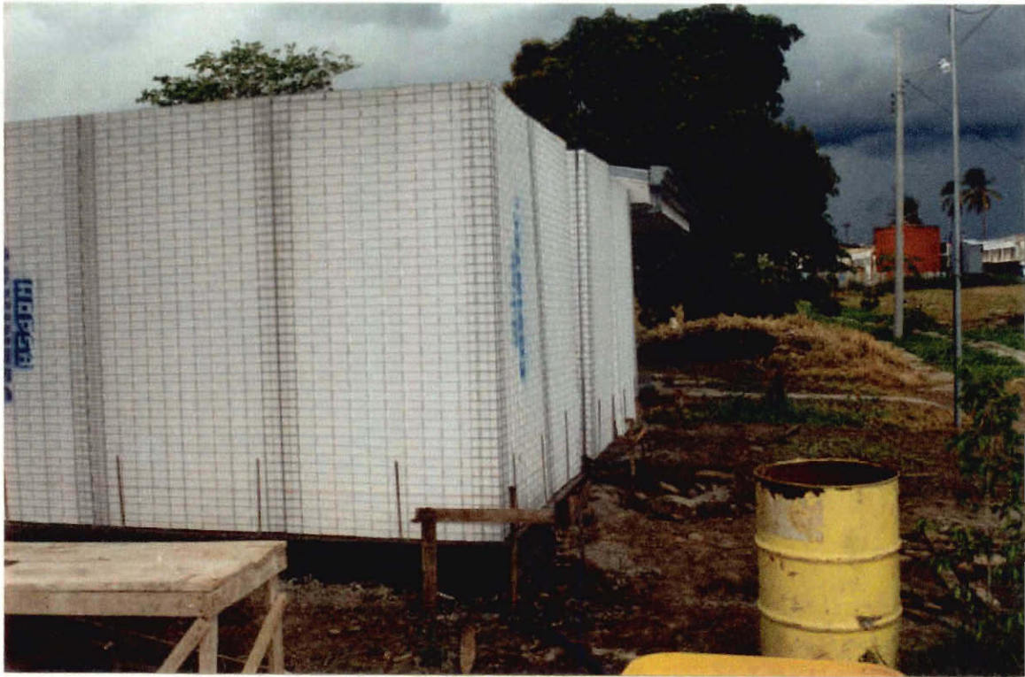
WALL CONSTRUCTED USING COVINTEC PANELS
