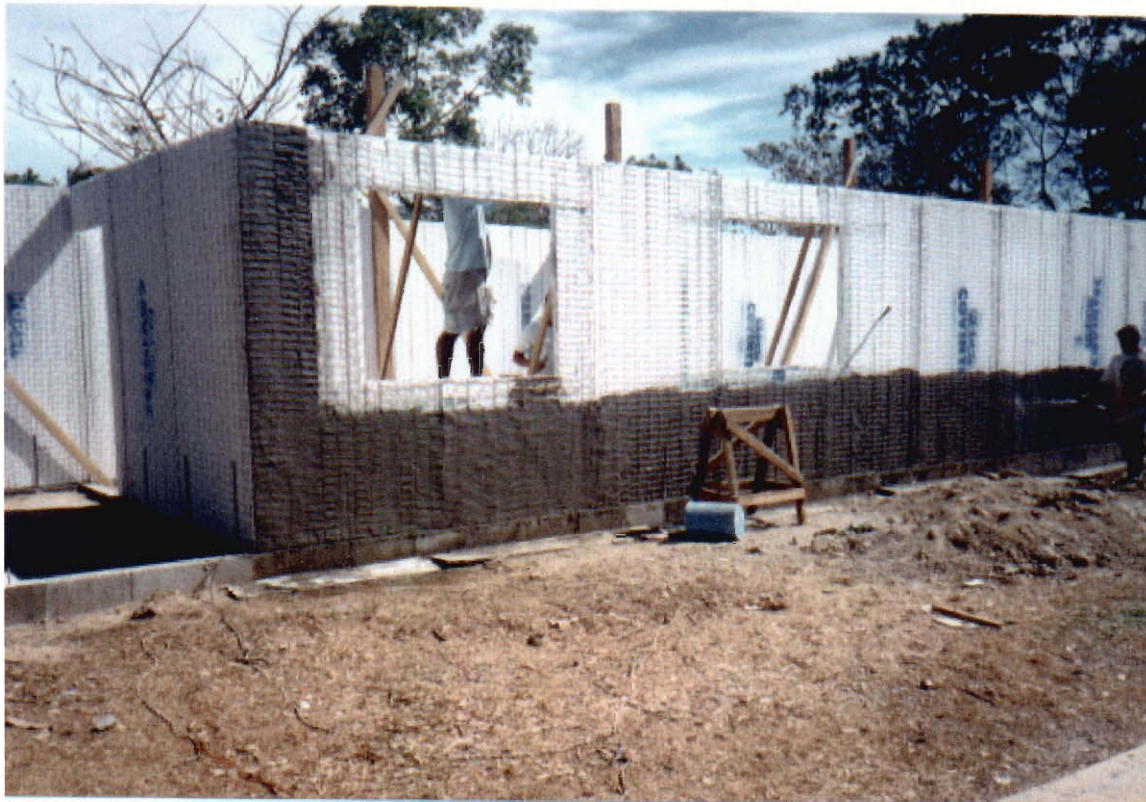
FIRST LAYER OF MORTAR BEING APPLIED TO THE WALL
