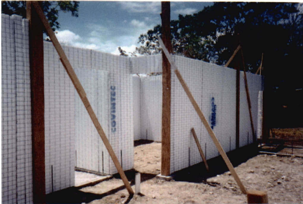
WALL CONSTRUCTED WITH COVINTEC PANELS
