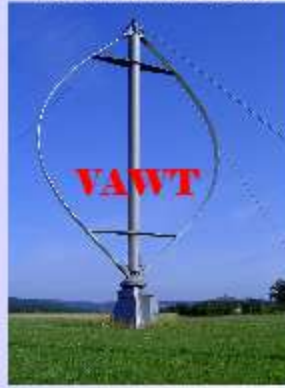
Vertical Axis Wind Turbine
