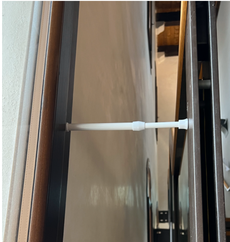
Figure 20: Tension rod testing between staircase and wall
