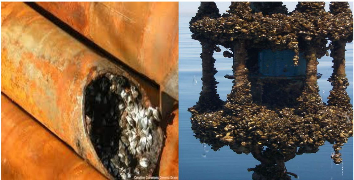
Figure 2.4 Zebra mussels cover a current meter (right) and clogged pipes (left) in Michigan (National Oceanic and Atmospheric Administration)
