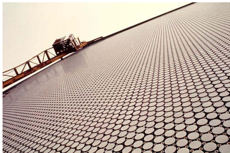
Fig. 5. 1. The Cobra Dane phased array system a) and the array face b) [52].
