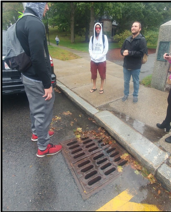
Above: Road Drain at corner of Institute Rd. and Boynton St.
