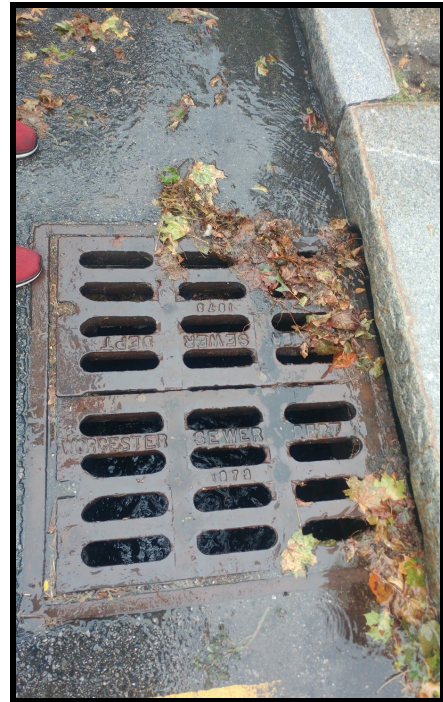
Above: Close up of Institute rd./Boynton St. Road Drain
