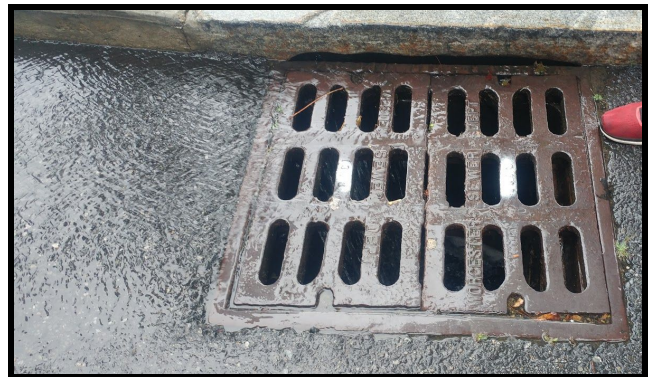
↑ Above: Up close view of road drain
