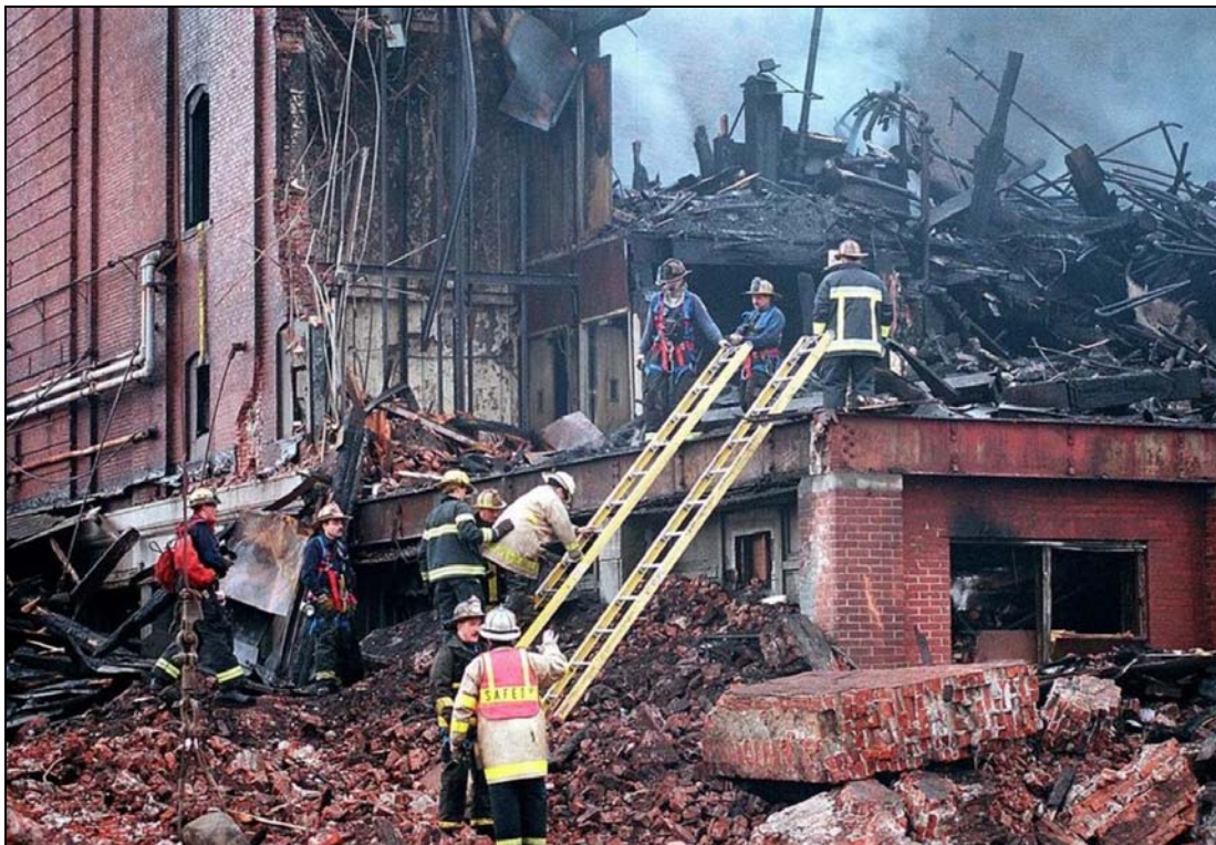
Image 9. Firefighters search through the rubble of the Worcester Cold Storage and Warehouse Co. structure. Teams of firefighters with specially trained dogs sifted through the charred wreckage and smoke drifted above the remaining three walls. (Photo by Paul Ferazzi, Telegram & Gazette , December 6, 1999)
