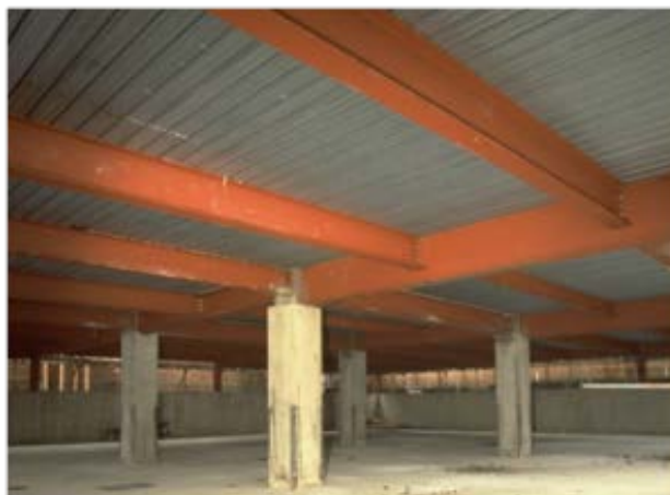
Figure: Fire Protecting Structural Steelwork (Fire Protection, 2014).
