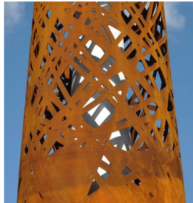
Figure 37 Perforated Metal Encasement (architectural Grille).
