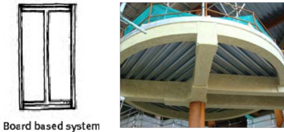
Figure:1 Fire protecting structural steelwork (Fire Protection, 2014).
