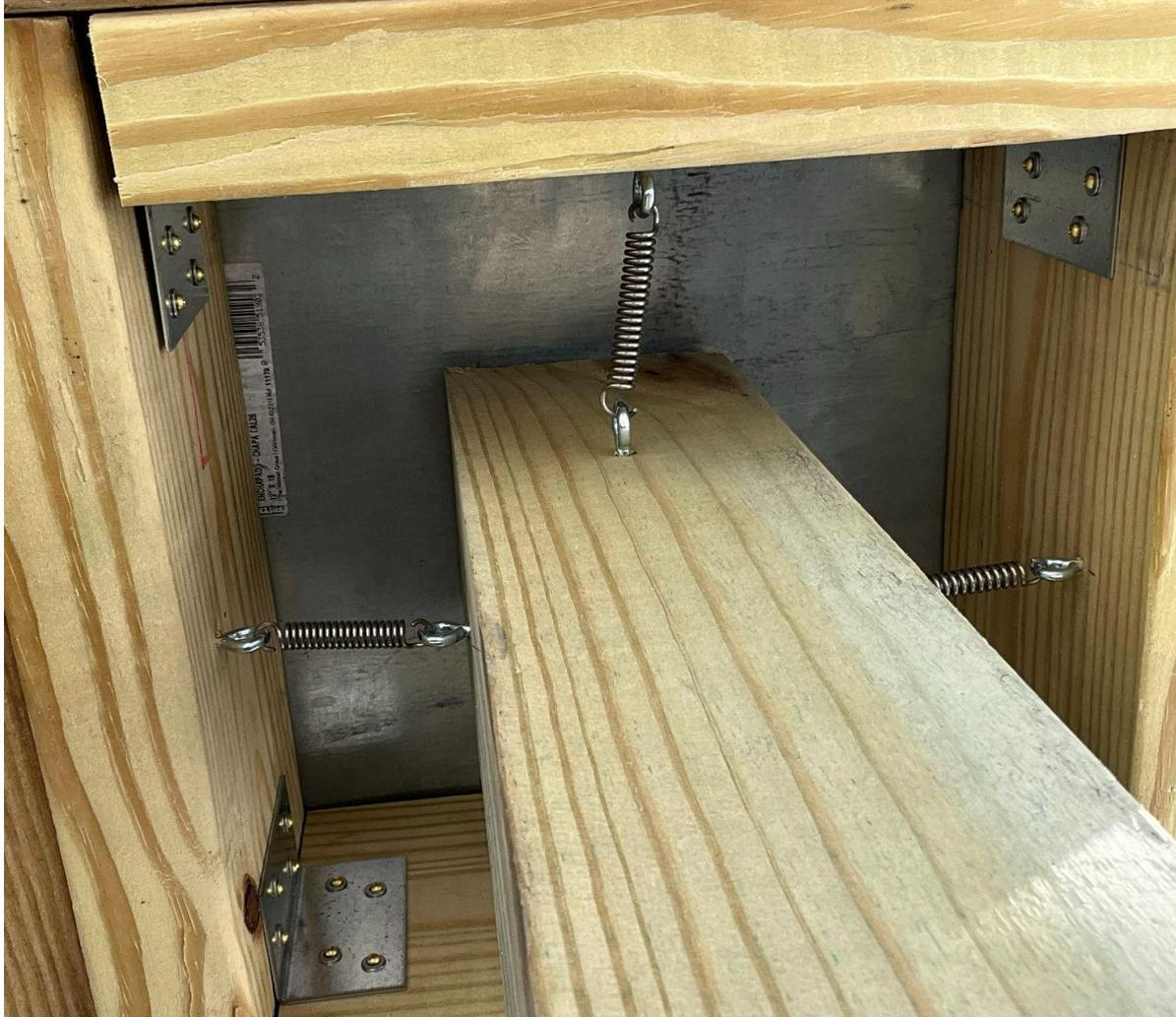
Figure 58: Underside of the initial prototype retrofitted to an existing dock
