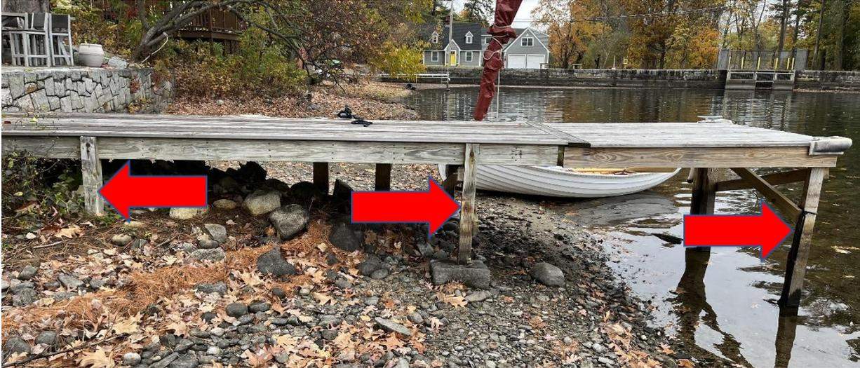
Figure 5: Fixed dock with light duty pilings in Westford, MA after the water was drawn down for the winter
