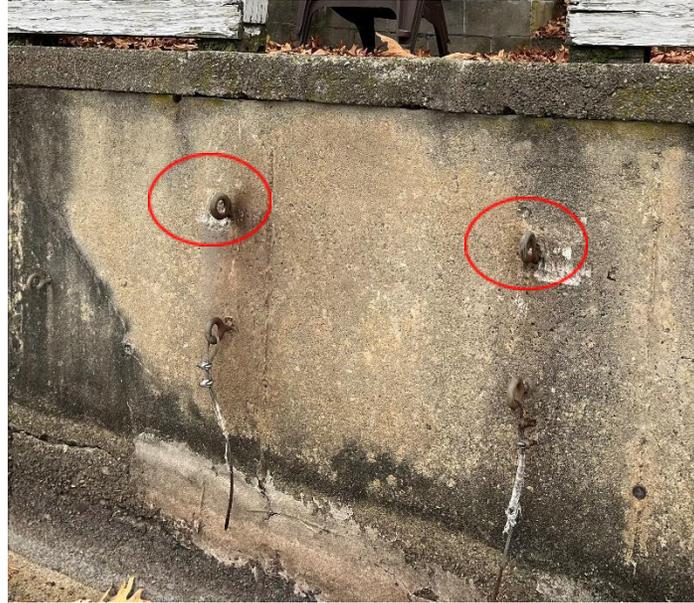
Figure 4: The eye bolts used to secure the floating dock to the shoreline in Westford, MA
