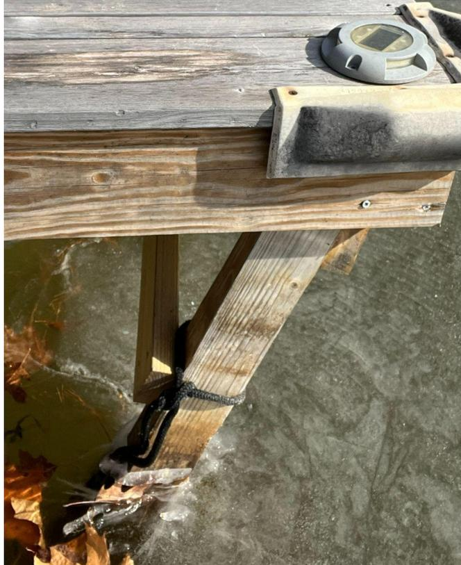
Figure 59: Normally fixed dock piling suffering permanent deformation
