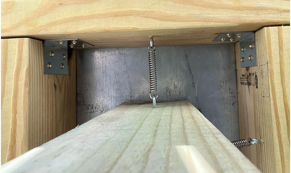
Figure 57: A stretched spring on the initial prototype retrofitted to an existing dock
