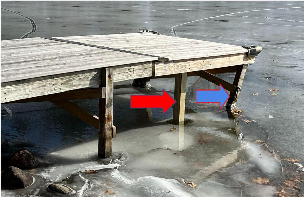
Figure 55: The initial prototype retrofitted to an existing dock
