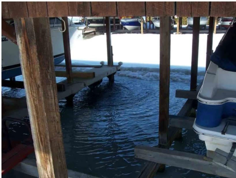
Figure 16: A dock bubbler being used to prevent ice freeze at a boathouse (Barbe, P., 2019, February 13)
