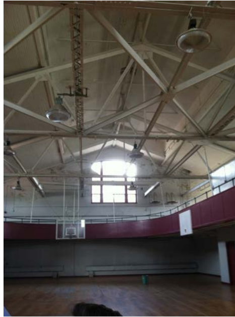
Figure 9: Interior View of Roof Showing Completed Construction
