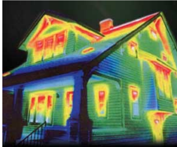
Figure 3 Thermal Image of a Typical Home (Thermography Proves Energy Efficiency of Post Frame Buildings, 2013)
