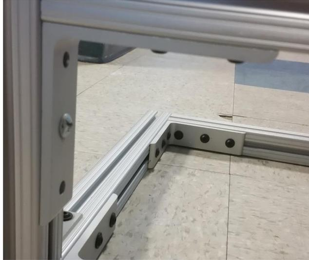
**Figure 5: L-brackets on Support Post**
