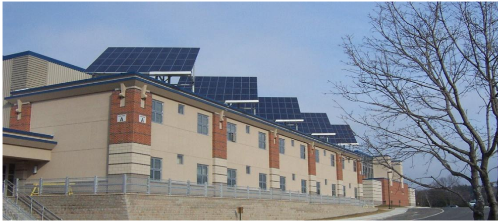
Figure 18: BVRHS Solar Panels (Blackstone Valley Regional Vocational Technical High School, 2009)
