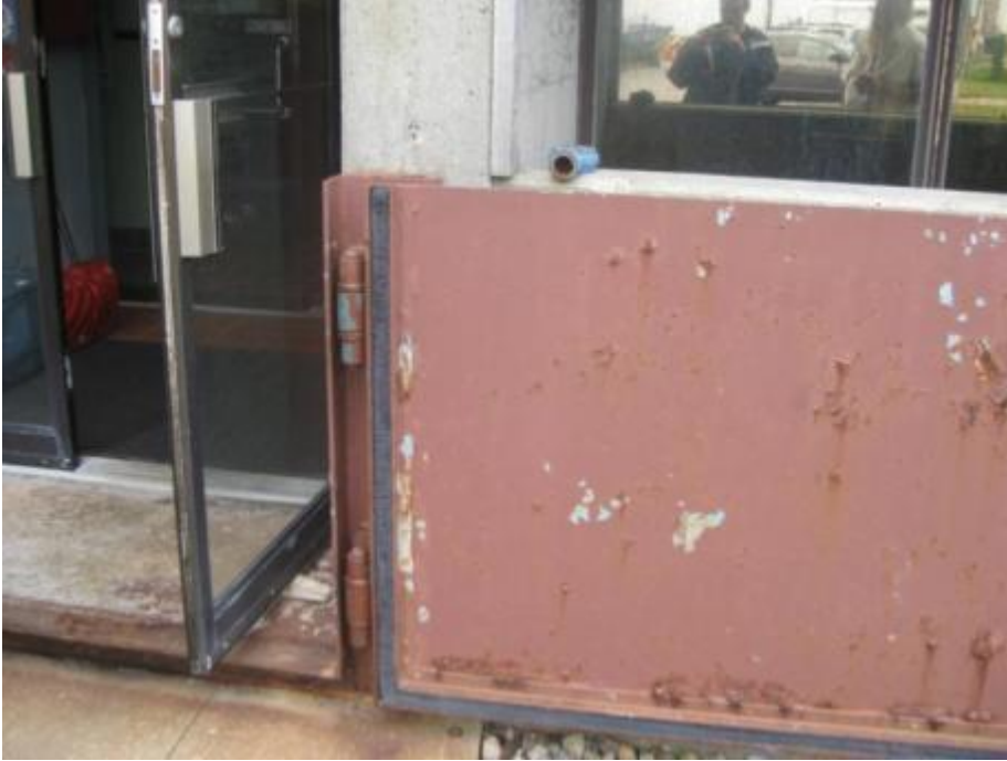
Figure F.1: Storm gate used at Hull Wastewater Treatment Facility
