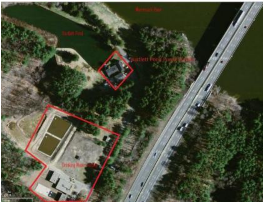
Fig G.1: Newburyport drinking water facility
