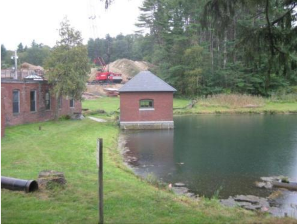
Figure G.2: Pump Station next to the Bartlett Spring Pond
